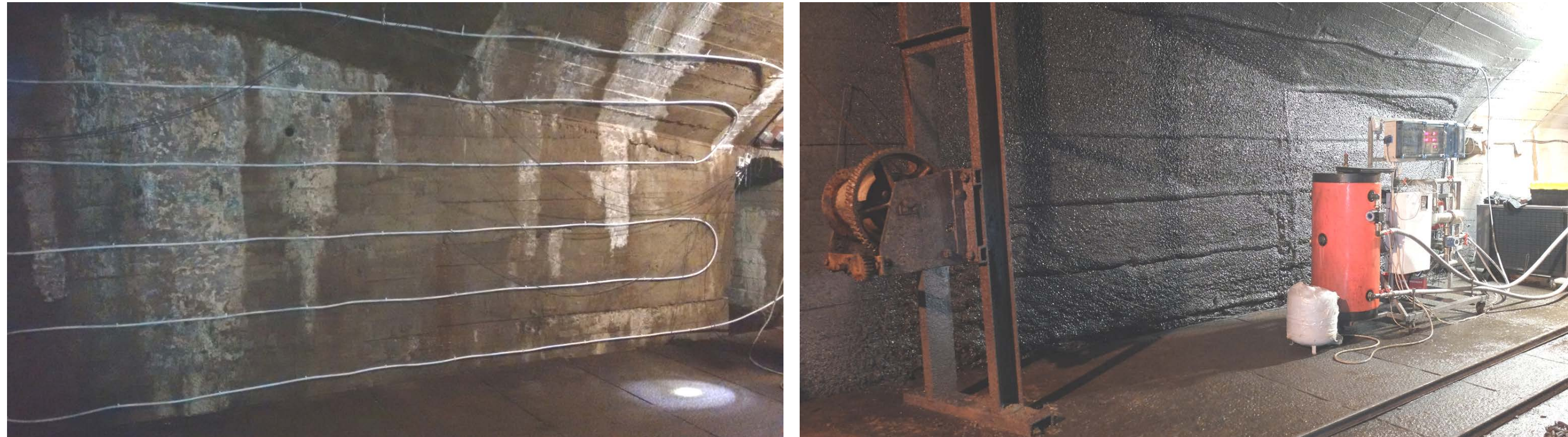
Left: PEX-Al-PEX tubes before TCM application; right: the heat exchanger with TCM and polyurea coating as water proofing.
